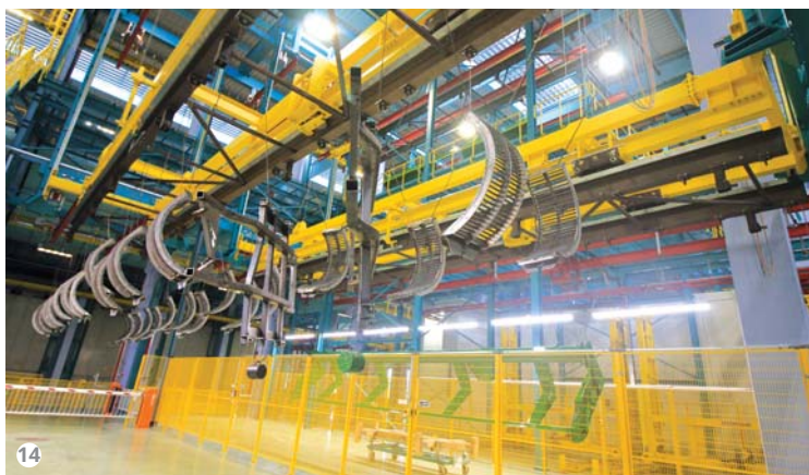
Figure 14: The two combined loading/unloading stations with an elevator of Agrostroy's Painting Line n. 3.
