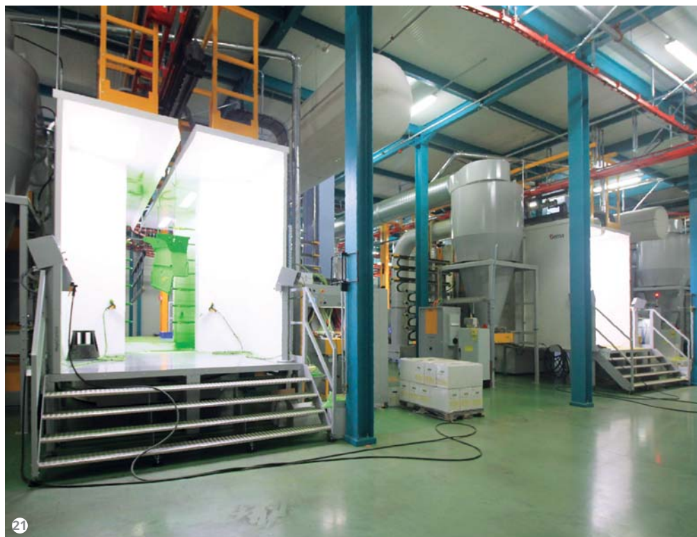
Figure 21: The powder coatings booths of the “plant within the plant”.
