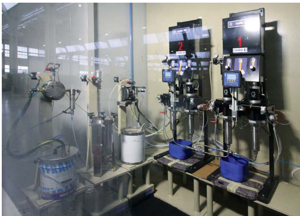
The coating management unit with Graco ProMix 2KE dispensers.
